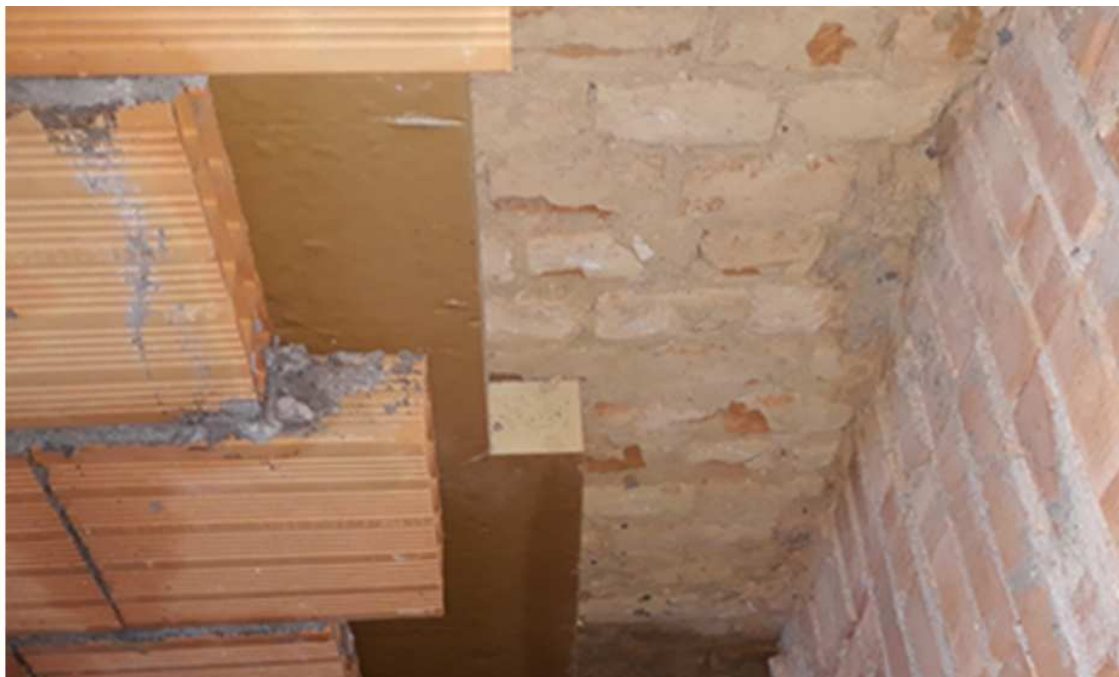
Fig. 18 – Internal counter-parks with an interposed insulating layer.
